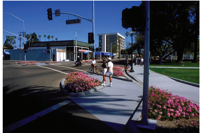
Figure C3. Small corner radii create slow turning speeds which allow motorists to meet the legal requirement to yield to pedestrians and bicyclists. Photo: Dan Burden
