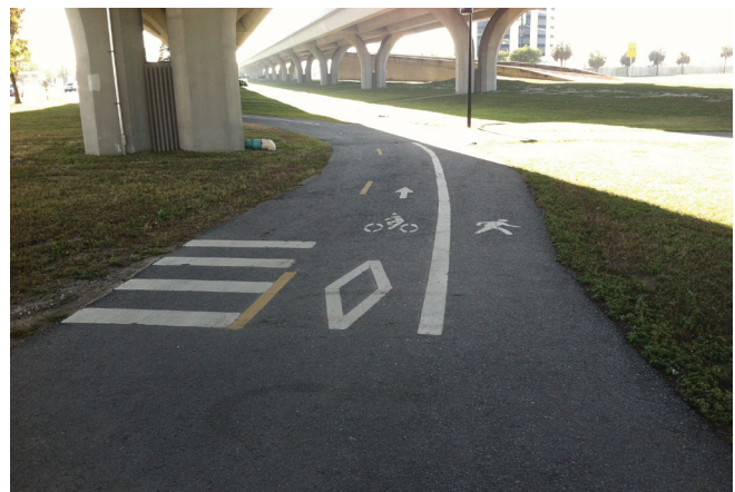
Figure C1. Pavement markings on a shared-use bidirectional path
