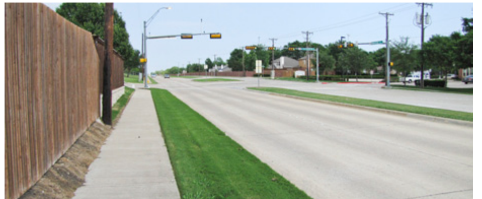
While this street accommodates 4’ wide sidewalks, narrow right-of-way along roadways makes providing an 8’ wide sidepath (the minimum width to accommodate cyclists and pedestrians) very challenging.
