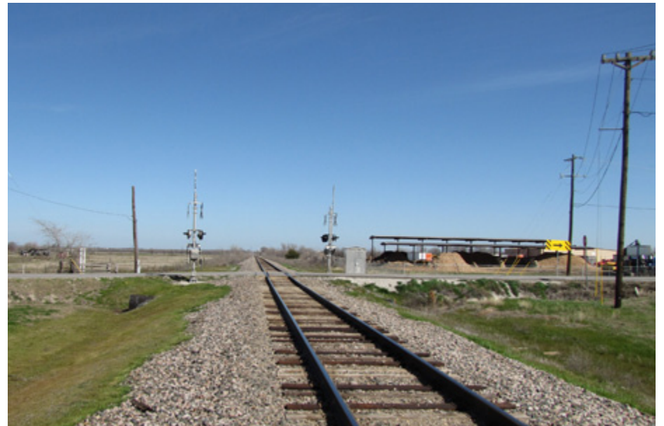
Looking north at the railroad crossing County Road 5.
