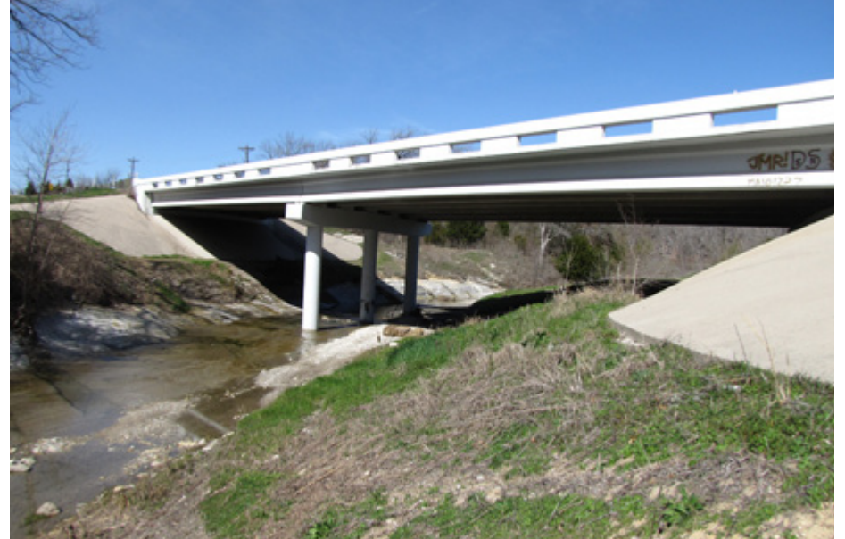
Looking northwest at the creek crossing under FM 1461.
