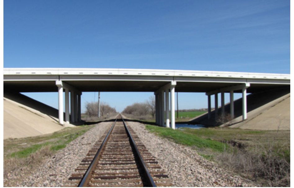
Looking north at the railroad crossing under US Highway 380.
