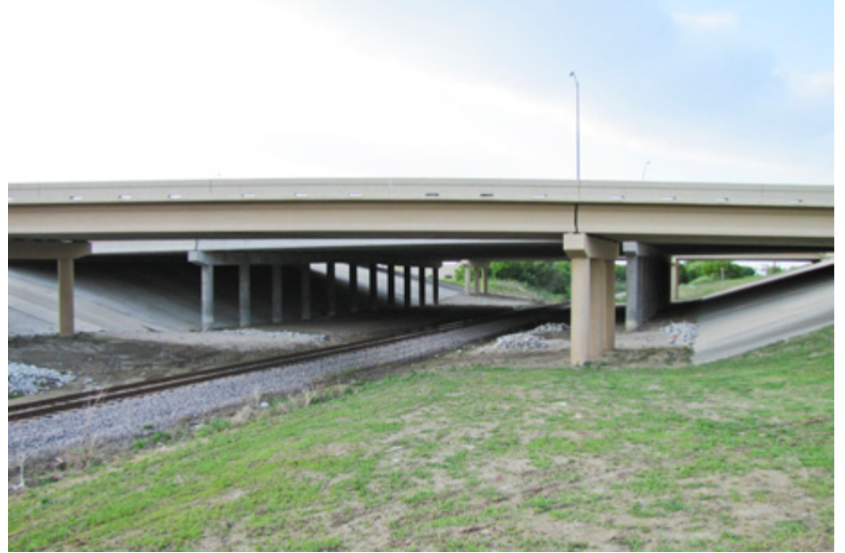
Looking north at the Highway 121 bridge over the Union Pacific railroad.
