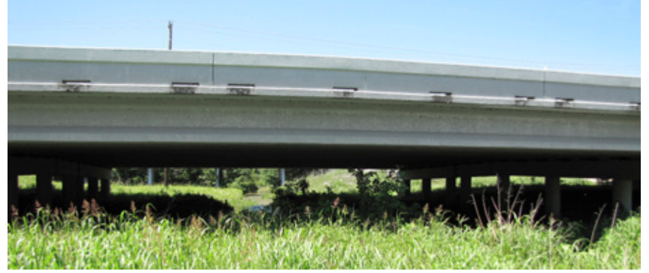
Looking north at the Highway 78 bridge.
