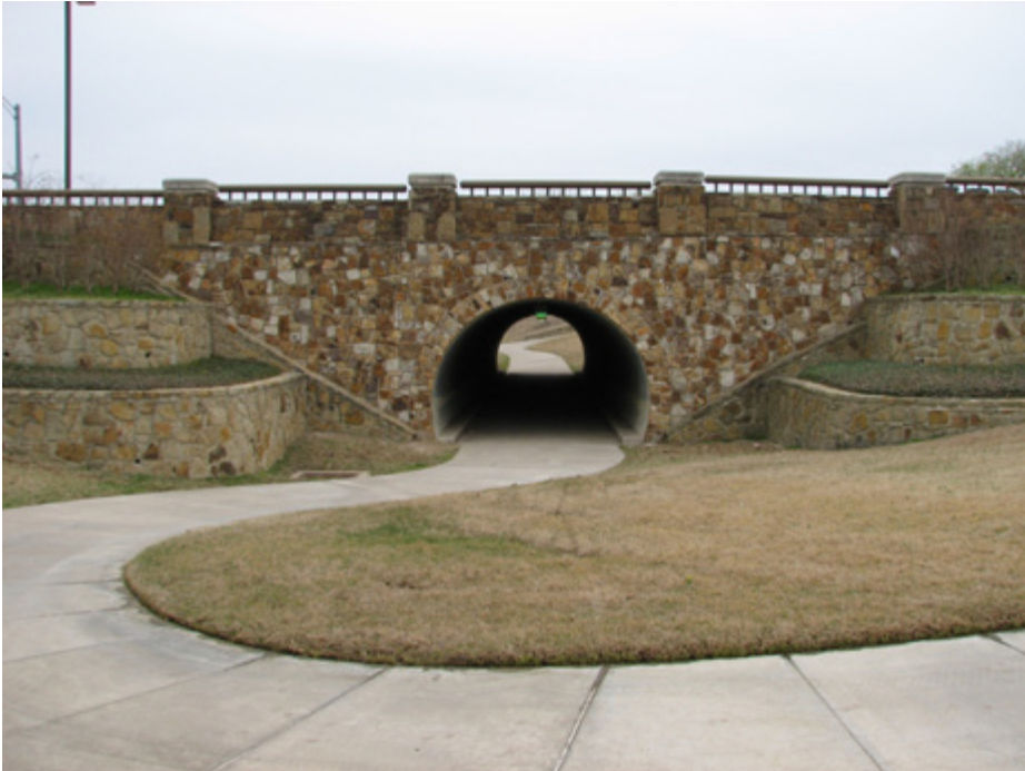
Grade-separated crossings minimize conflicts between trail users and automobiles, but are more costly to construct. Retrofitting such a crossing under an existing roadway can be prohibitively expensive.
