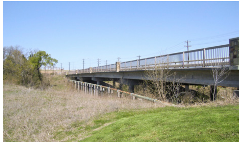
Looking northeast at the Custer Road bridge. The sewer pipeline is visible below the bridge.
