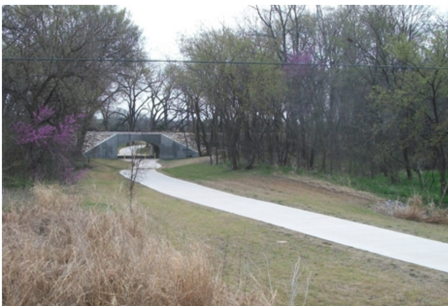
The City of Allen was able to work with DART to provide a trail underpass under the DART rail line.
