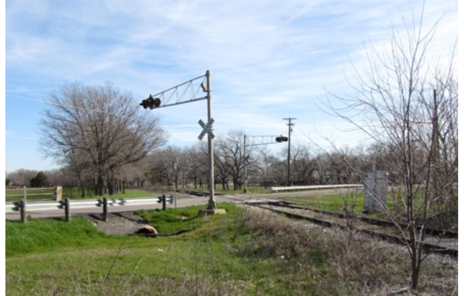
Looking northeast at the Country Club Road railroad crossing.
