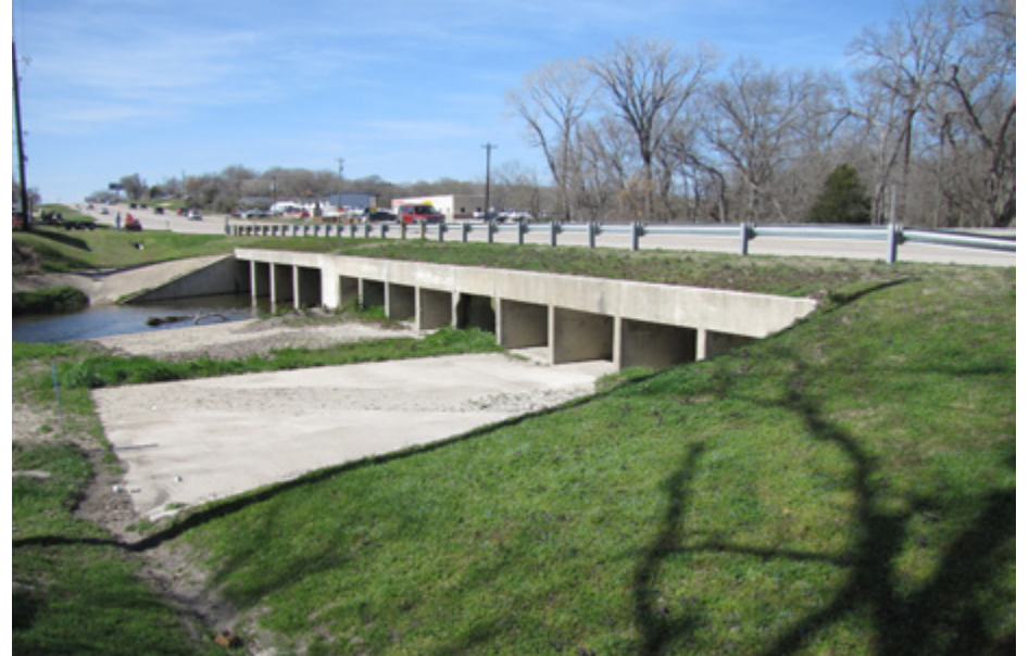
Looking northwest at the Highway 380 culvert over Big Branch Creek.
