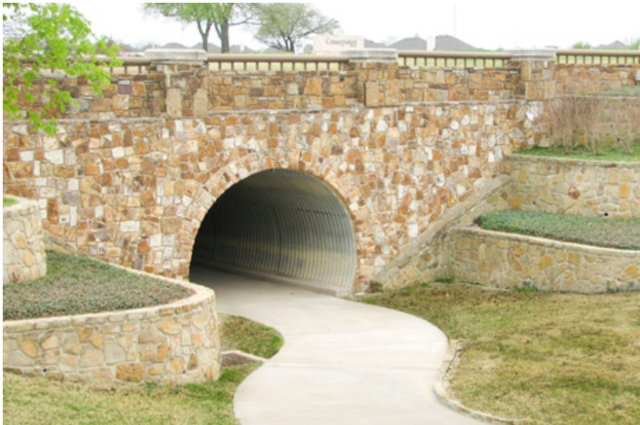
Roadways also present barriers for trails in many cases. McKinney has proactively accommodated trail crossings by building trail underpasses when new roadways are constructed.
