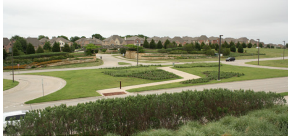
At-grade trail crossings require careful consideration of traffic speeds and volumes, sight-lines, and trail user volumes to ensure a safe crossing design.
