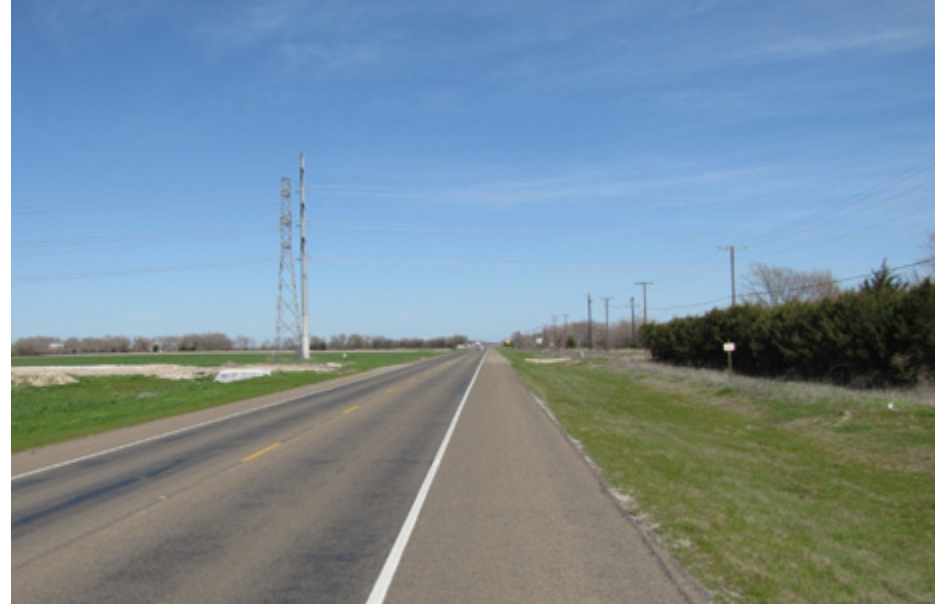
Looking south along Highway 5. The construction on the left of the image is the west-bound frontage road of the future Outer Loop. The railroad is parallel to the highway behind the row of trees on the right side of the image.
