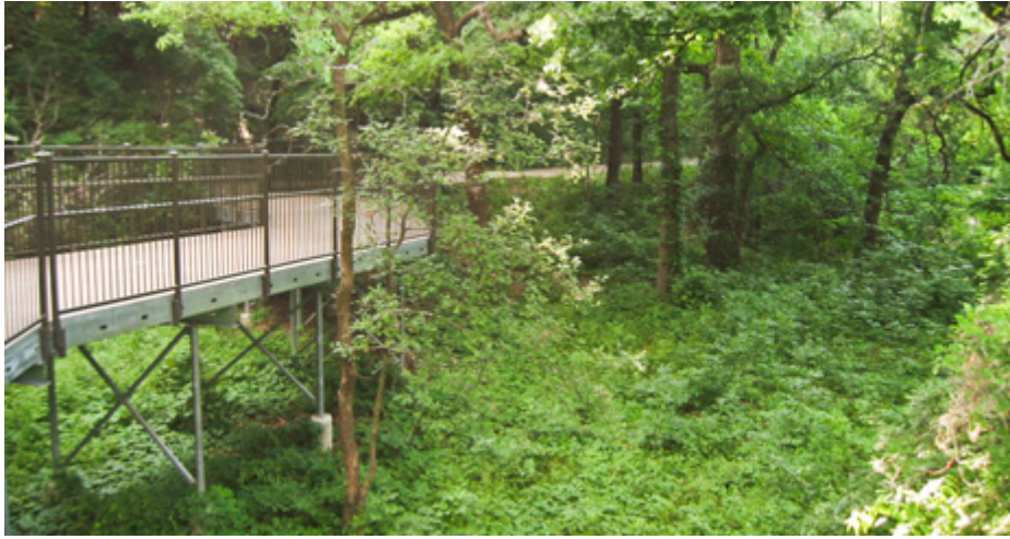
Trails along creek corridors can provide significant challenges in terms of drainage, topography, and erosion. Shady Brook Trail in Plano utilizes boardwalk/bridge structures to address these issues.
