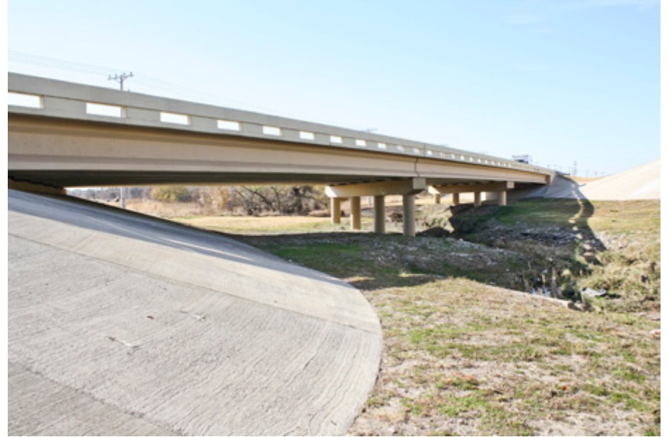
Looking southwest at the State Highway 121 bridge.
