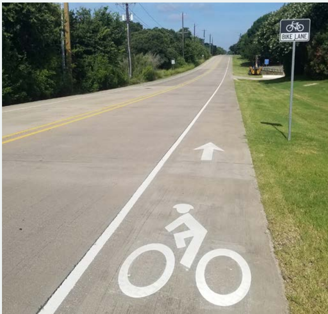
Clear signage and pavement marking to indicate the portion of the roadway that bicyclists can utilize alerts motorists of the potential presence of bicycles.
