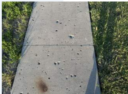
The paths are only four feet wide and are in need of maintenance and repairs.
