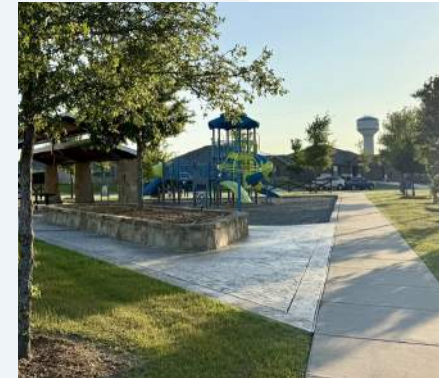
Playground, raised planter, and shade structure at Magnolia Pointe.
