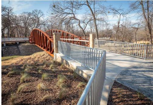
side of a trail structure should be 4' higher than the trail surface. Railing ends should be angled downward and flared away from the trail at both ends to prevent injury. Railing rungs should be horizontal in orientation so as not to catch bicycle handlebars. The bottom rung of a railing should be 4" from the finished trail grade. Trail safety railings should also be in accordance with the 2015 International Building Codes.
