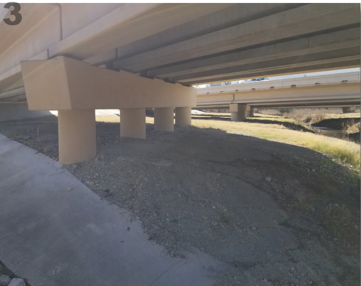
3 UNDER HWY 75 BRIDGE CROSSING LOCATION LOOKING WEST
