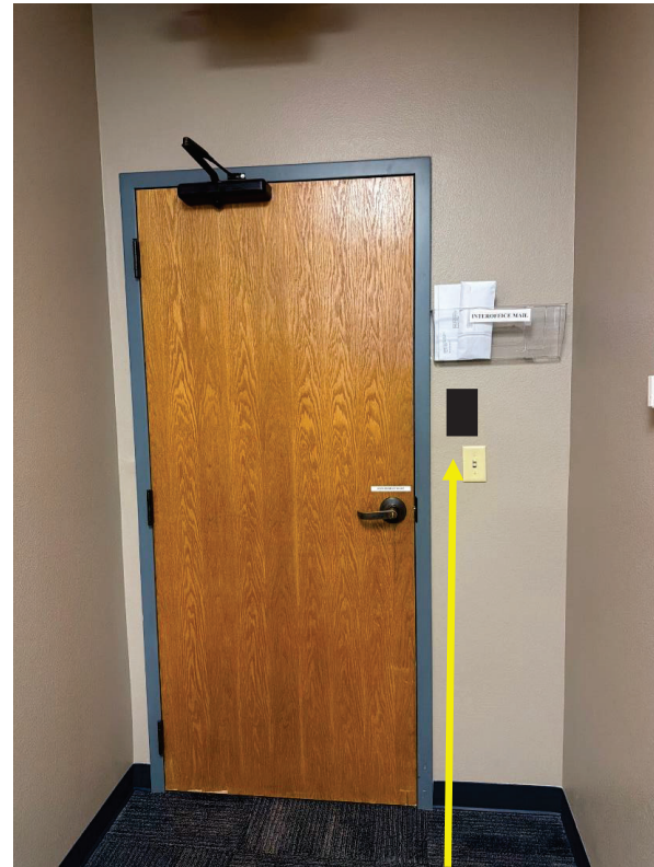
Constable PCT 4 door Inside door Install card reader
