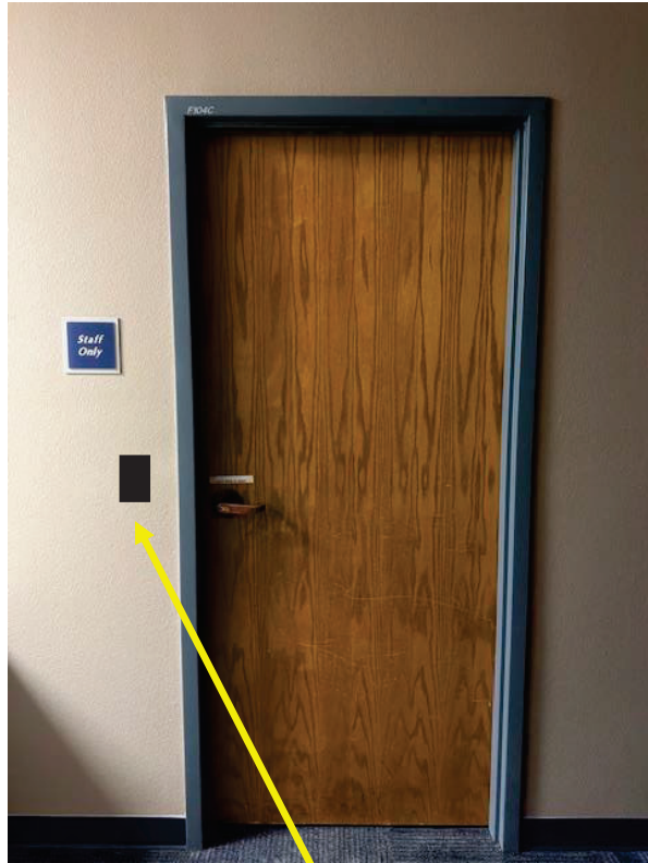
JP 4 Courtroom Door Install card reader Inside & Out
