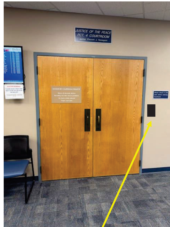
JP 4 Front Courtroom Door Install card reader Inside & Outside
