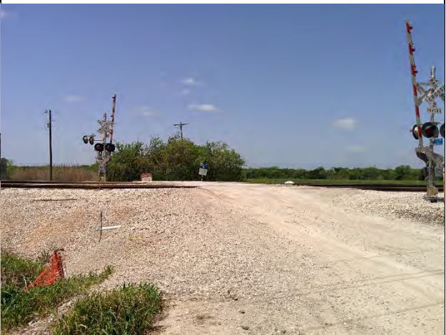
#4 Railroad Crossing of UPRR
