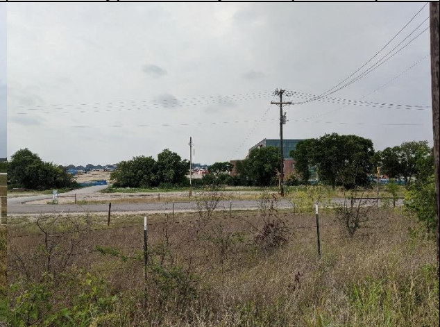
#4 New Construction south of Hackberry Cir.
