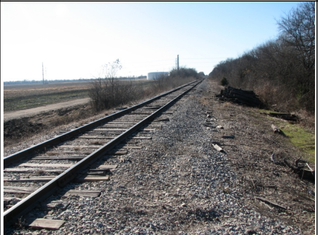
#4 DART owned railroad adjacent to SH 5
