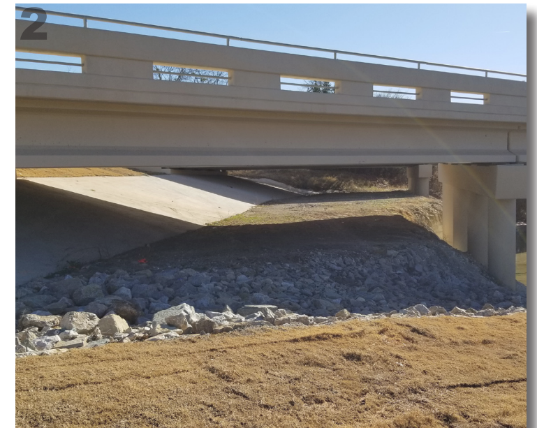
121 SAM RAYBURN HWY OVERPASS LOOKING SOUTHEAST
