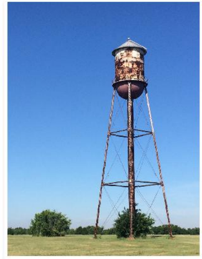
Historic Elevated Storage Tank at J.M. Caldwell, Sr. Community Park
