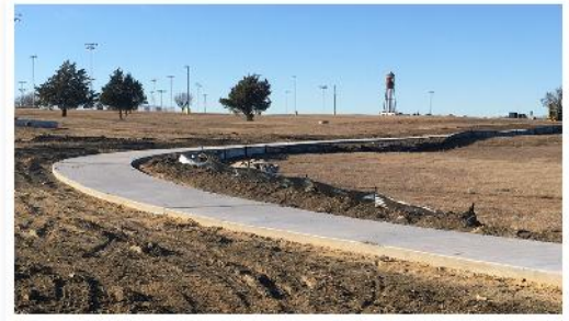
Eight Foot Wide Trail Construction at J.M. Caldwell, Sr. Community Park
