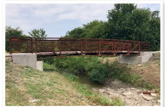
Pedestrian Bridge at J.M. Caldwell, Sr. Community Park
